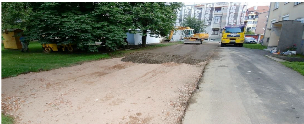
Figure 3: Incorporation of recycled aggregate – example of good practice (Source: Author's elaboration of dana)
